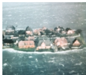
Flooding in more recent years
