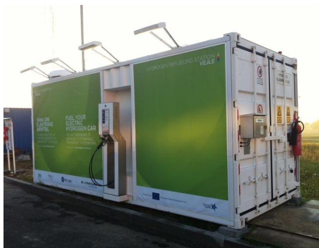
Figure 5: Green Network's HyTrEc-funded demonstration of containerised HRS (Source: HyTrEc-Partnership)
