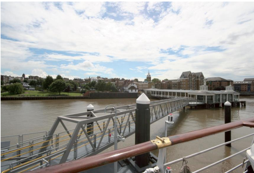
The new pontoon landing at Gravesend
