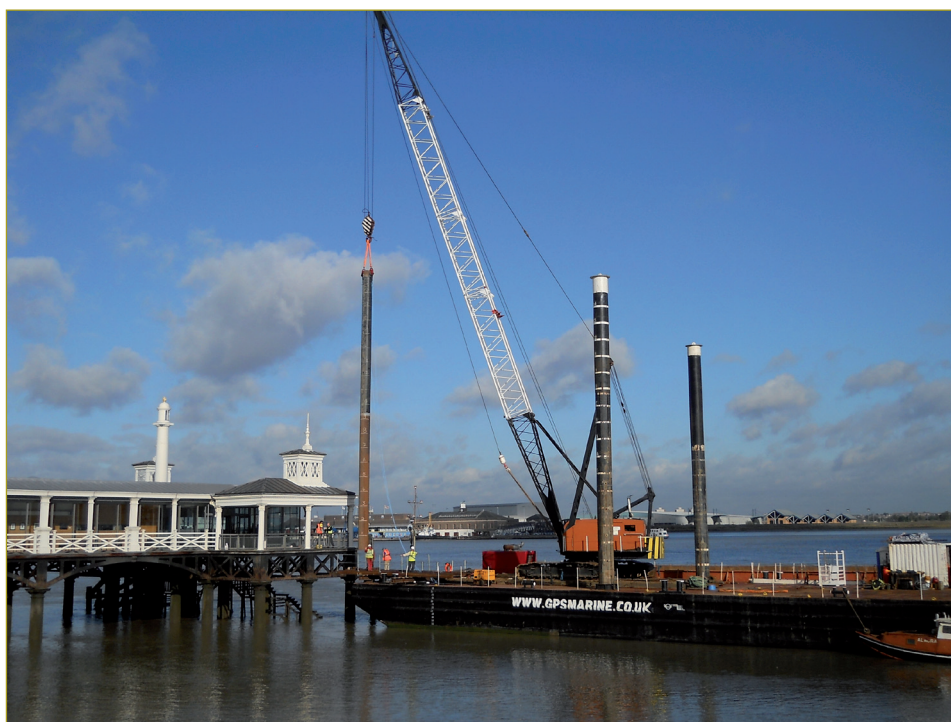
Pitching piles - the public were kept informed at each stage of construction
