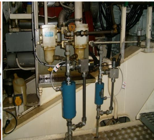
Fig.6: flow meter installation (blue tubes)
