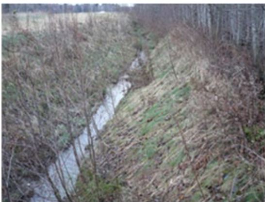
Figure 6: Ditch with runoff from balancing pond – to be expanded as a constructed wetland
