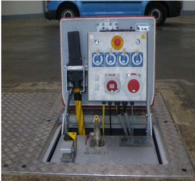
Figure 2, Under floor Power Station
