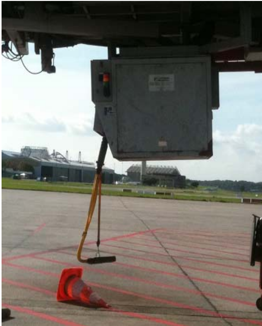
Figure 5, Electrical Power Supply (Gangway)
