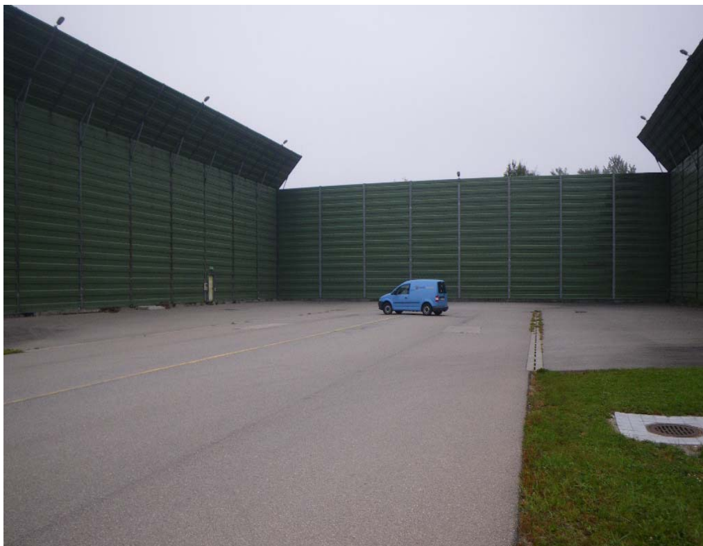
Figure 6, Noise Protection Hangar (U-shaped), Investment € 1,5 Mio
