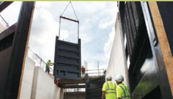
Liverpool Canal Link Lock Gates Installation (UK)
