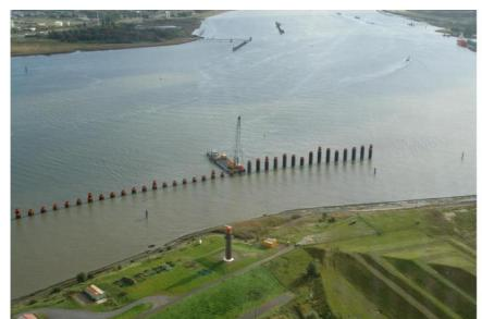
Figure 18: Construction of current deflecting wall at Deurganckdok (<u>http://www.hye.be/nl/news/show/one/9/</u>)
