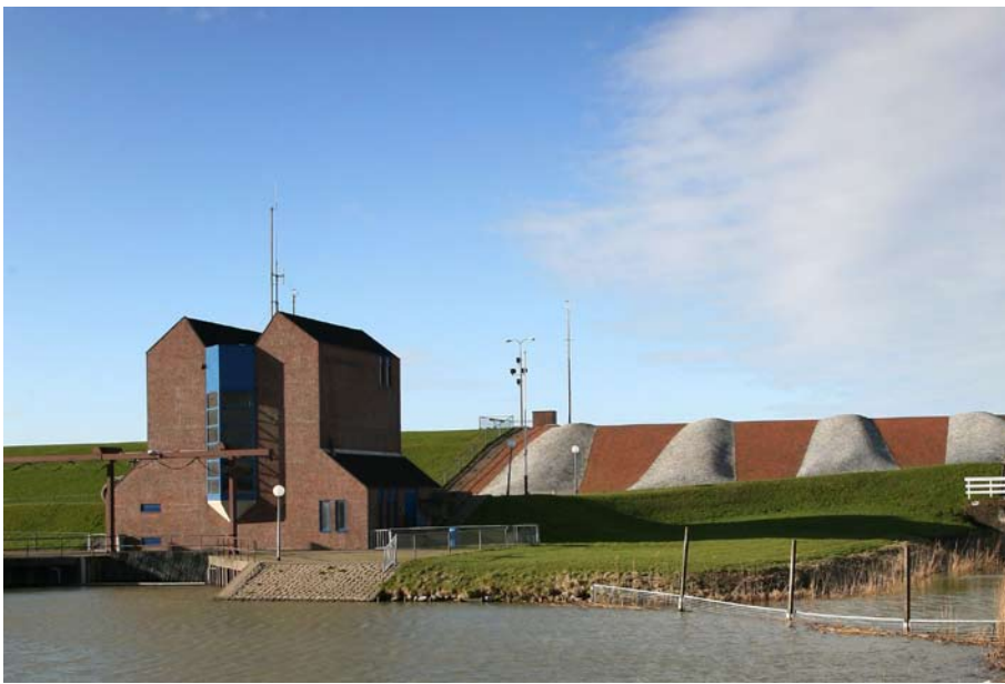
Pumping station Noordpolderzijl (the Netherlands), one of the three fish pass projects.
