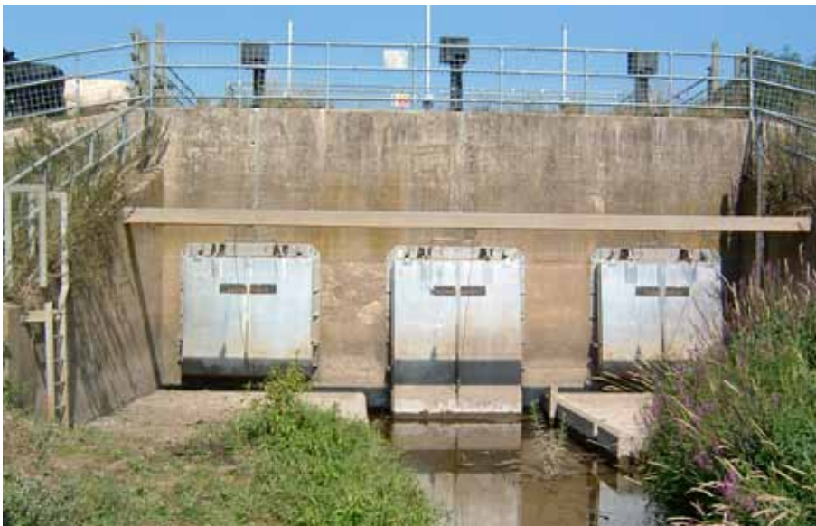
Deerhurst Drain outfall
