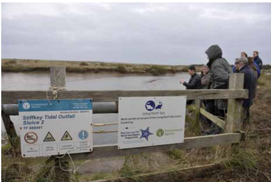
LNS Pilot project: Stiffkey tidal outfall sluice (UK)
