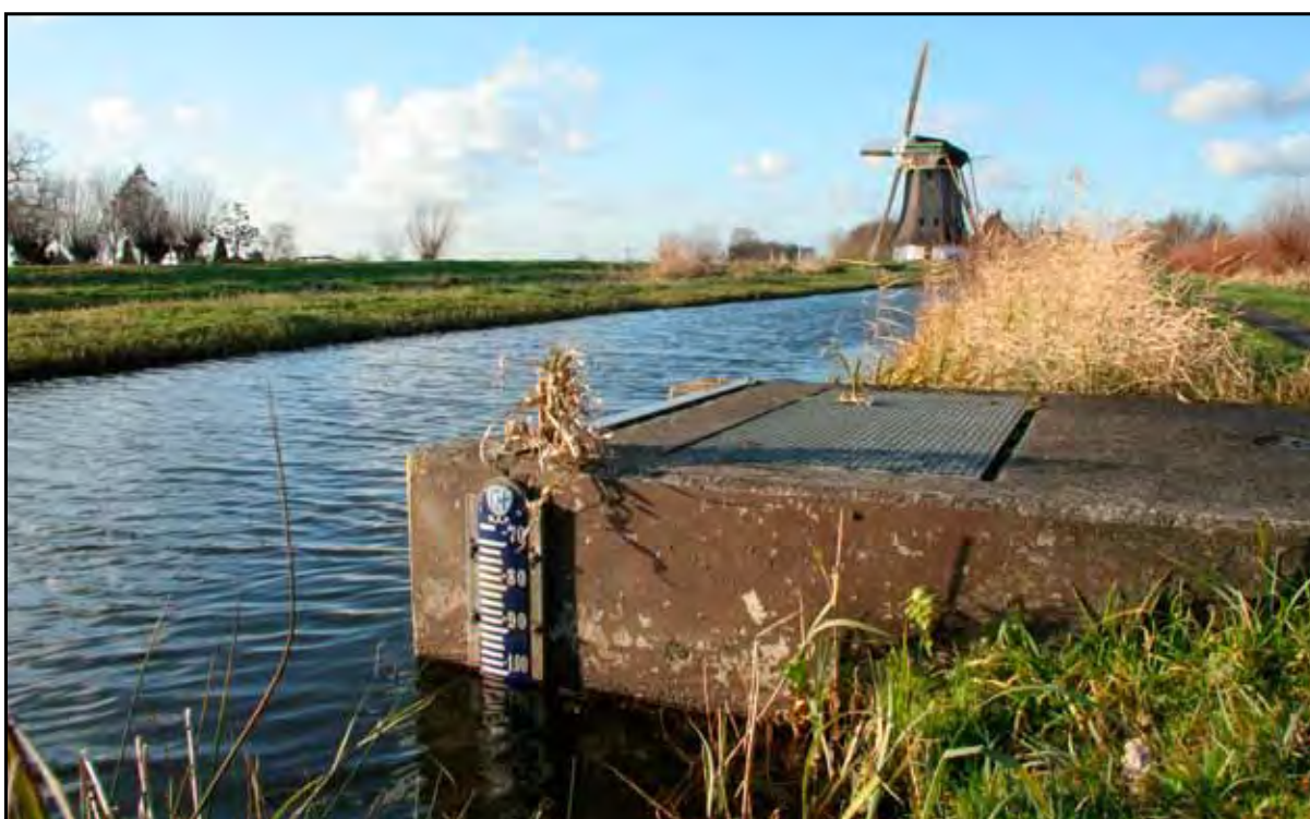
Pumping Station Naardermeer NL. A traditional windmill with water wheel is still being used to control the water level
