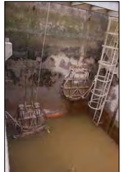
Round cast iron flap gates, Addlingflet drain, River Trent, UK, passive operation
