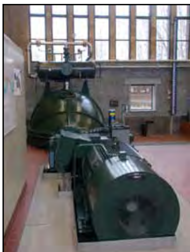
Examples of diesel powered pumps typical of those installed in tidal pumping station throughout the NSR in a period 1930-60s. Many of these pumping stations use centrifugal or screw pumps, which cause significant mortality to fish if attempting passage. East Stockwith Pumping station River Idle, UK
