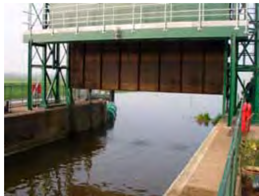
Tidal door being lifted open on incoming tide as part of LNS Fish Migration Day, River Nene, UK
