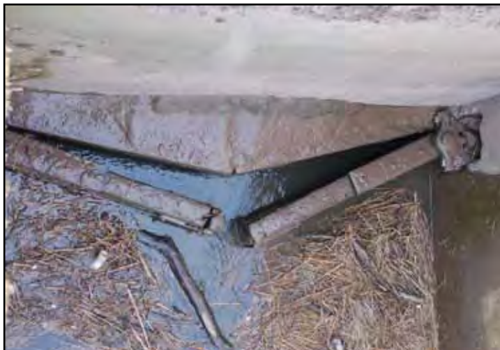
Pointing doors, tidal Trent, UK, passive operation
