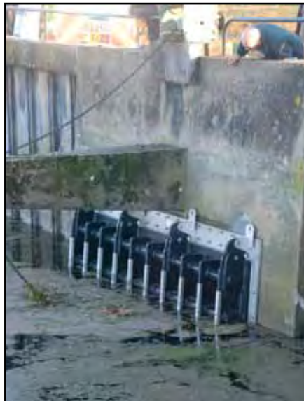
Tidal flap gate made from modern HDPE plastic, offers a light gate with better sealing over a wooden gate, light weight materials can be beneficial for fish passage as less water pressure is need to open them, but HDPE gates also seal better and have less opportunity for leakage that can make fish passage harder.
