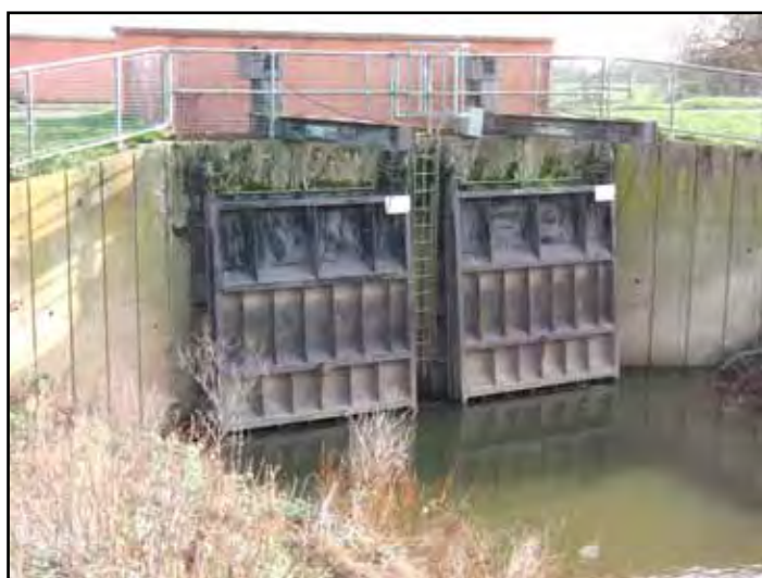
Metal fluvial flap gates on the end of the River Chelt, UK, Passive Operation
