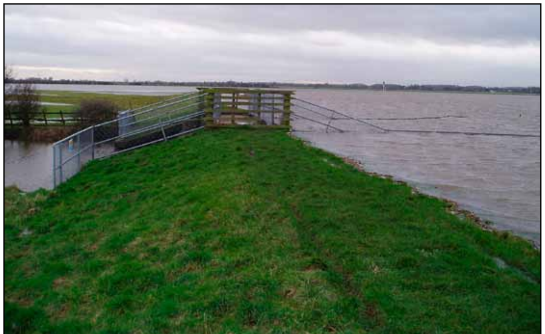
Fleet Outfall, River Trent UK, in flood conditions showing how tidal defences disconnect the river from its floodplain
