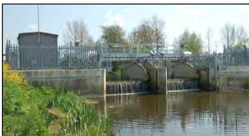
Metal fluvial flap gates on the end of the River Chelt, UK, Passive Operation
