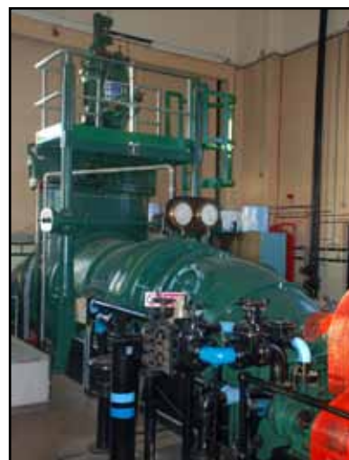
Examples of diesel powered pumps typical of those installed in tidal pumping station throughout the NSR in a period 1930-60s. Many of these pumping stations use centrifugal or screw pumps, which cause significant mortality to fish if attempting passage. East Stockwith Pumping station River Idle, UK
