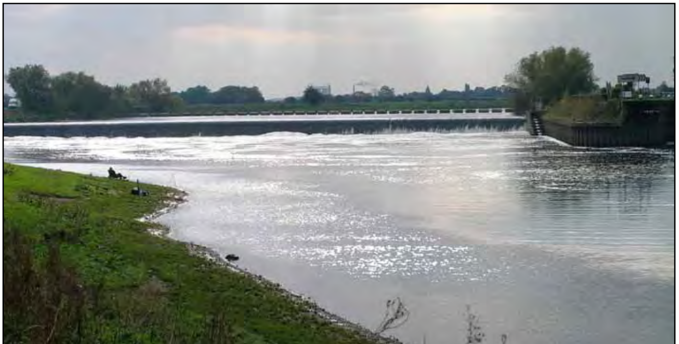
Cromwell Weir at head of tide on the River Trent, UK. This weir forms the first barrier to fish migration unless inundated by spring tides
