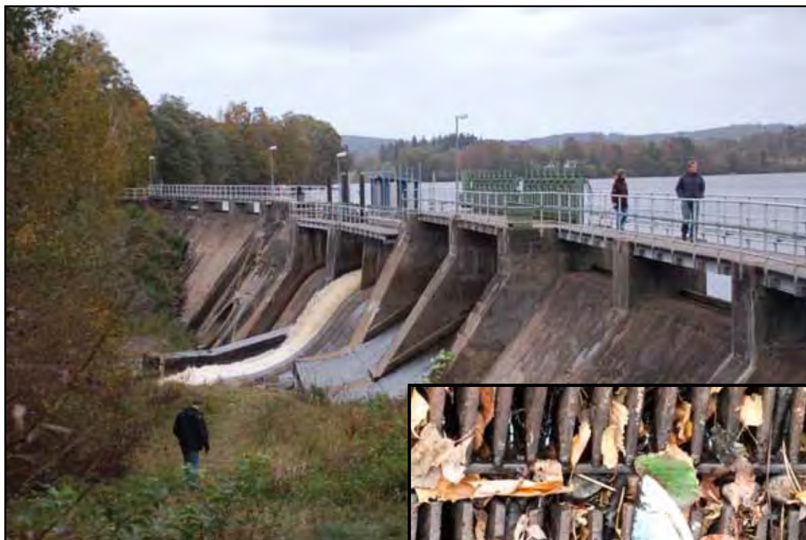
Atrafors Hydropower Dam, Sweden and entrained bream on intake screen to hydropower plant
