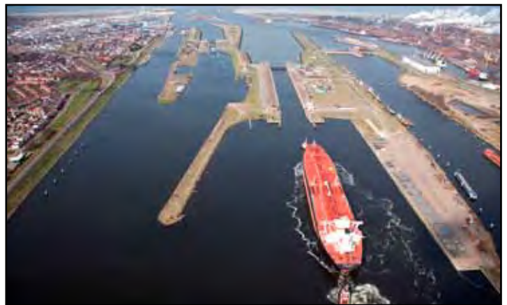
Tidal barrier, Noordzeekanaal IJmuiden, Netherlands. Includes locks, siphons for gravity discharge and the largest pumping station in the Netherlands (max. 750 m 3 .s -1 )
