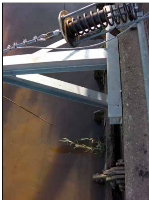
Retarder spring attached to winch cable of wooden flap gate on the River Trent, UK. The spring compression extends the period of the gate remaining open on an incoming tide to increase opportunity for glass eel migration from tidal to freshwater habitats
