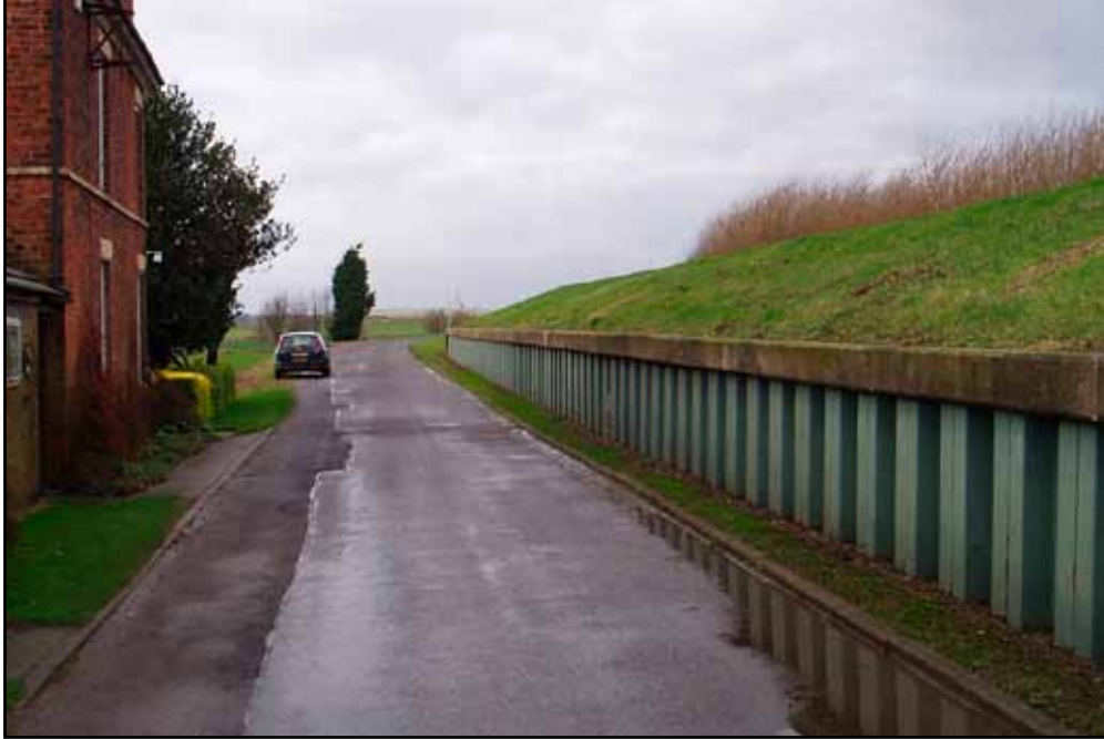
Flood bank on River Trent, UK showing how much higher the river is in relation to the surrounding land
