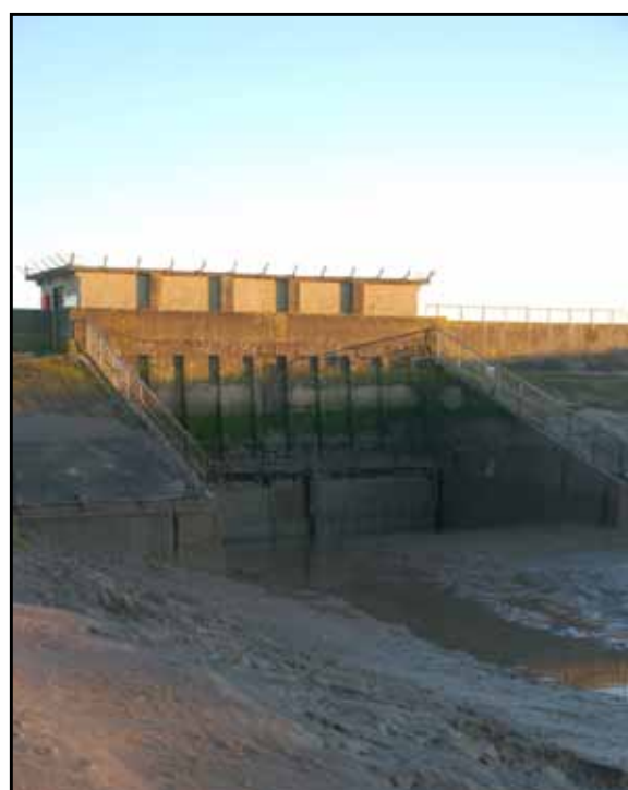
Large gravity controlled tidal flap gates, Huntspill Outfall, Somerset, UK, passive operation
