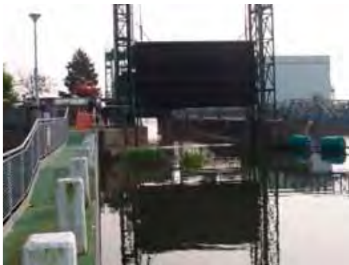
Tidal door being lifted open on incoming tide as part of LNS Fish Migration Day, River Nene, UK
