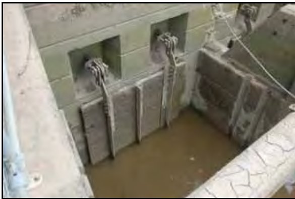
Wooden tidal flap gates, River Trent UK, passive operation
