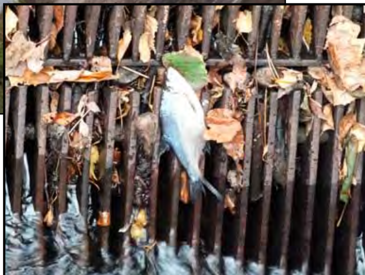
Atrafors Hydropower Dam, Sweden and entrained bream on intake screen to hydropower plant
