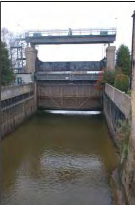
Tidal gate on the River Nene, Cambridgeshire, UK. This can be lowered to isolate tributary during tidal surges or fluvial flood event, mechanical operation
