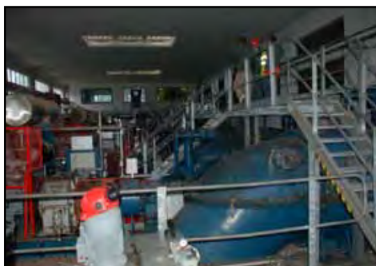
Inside Keadby Pumping Station on the River Trent, UK. Showing the amount of pumps needed to prevent flooding during storm events
