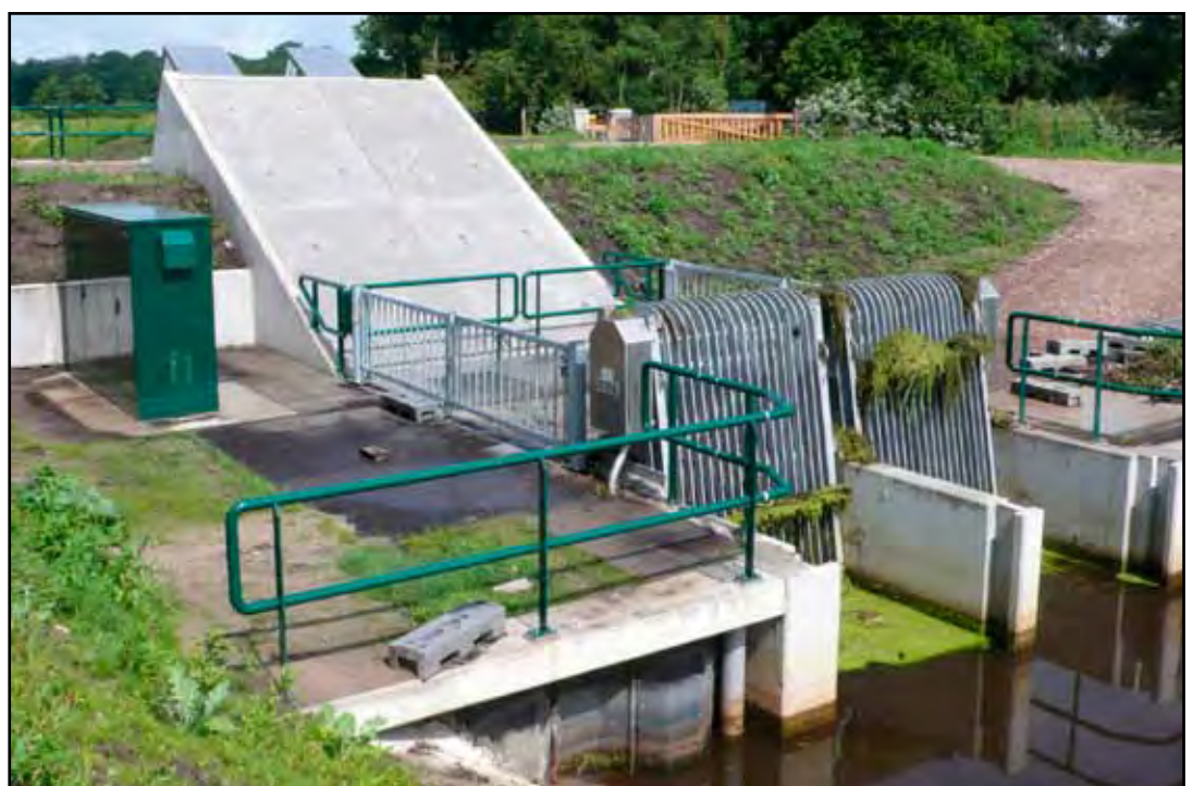
Pumping station Ennemaborgh (The Netherlands), fitted with two specially adapted fish friendly Archimedes screws
