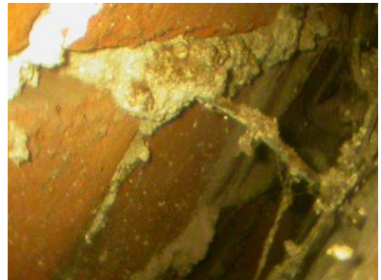
Endoscope photo of cavity with masonry tie
