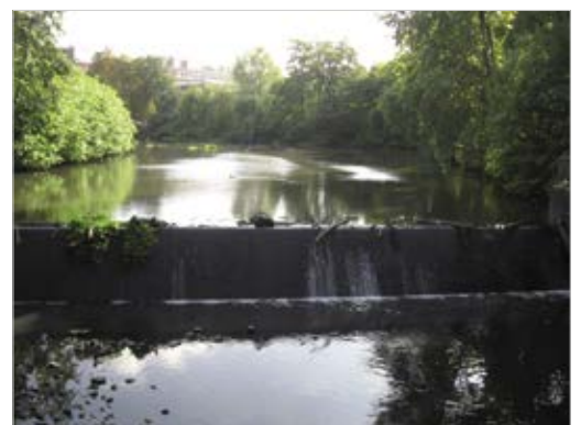
Ponded sections in the River Wandse network are not consequently optimized to retain severe floods and pose demand for restoration of aquatic animal passage.
