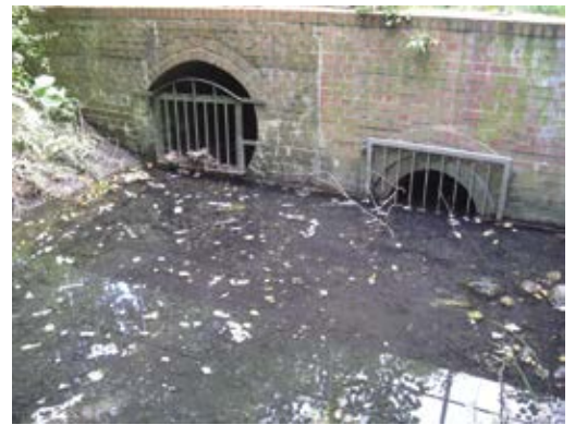
Fast run-off from the rainwater canalisation dominates the flooding events following short and intense rainfall, and is associated with considerable sediment, nutrient and pollutant loads.
