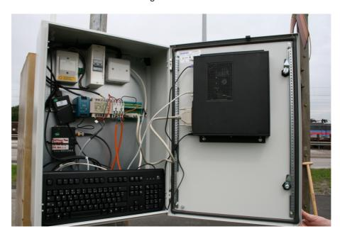
Each read point consists of an RFID reader, an RFID reader antenna, a GPRS modem and two axle readers installed in the track. The read point in the Port of Göteborg also includes a PC as indicated in the picture above.
