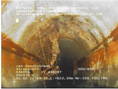
Figure 2.2 Picture of sewerage Wielwijk from a recent video inspection
