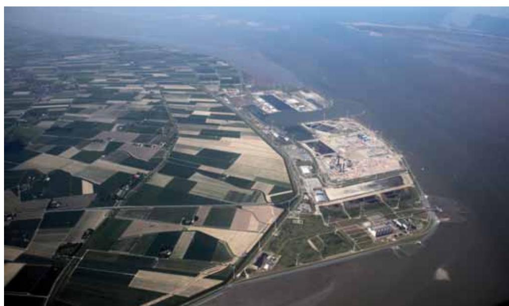
Aerial view of Eemshaven
