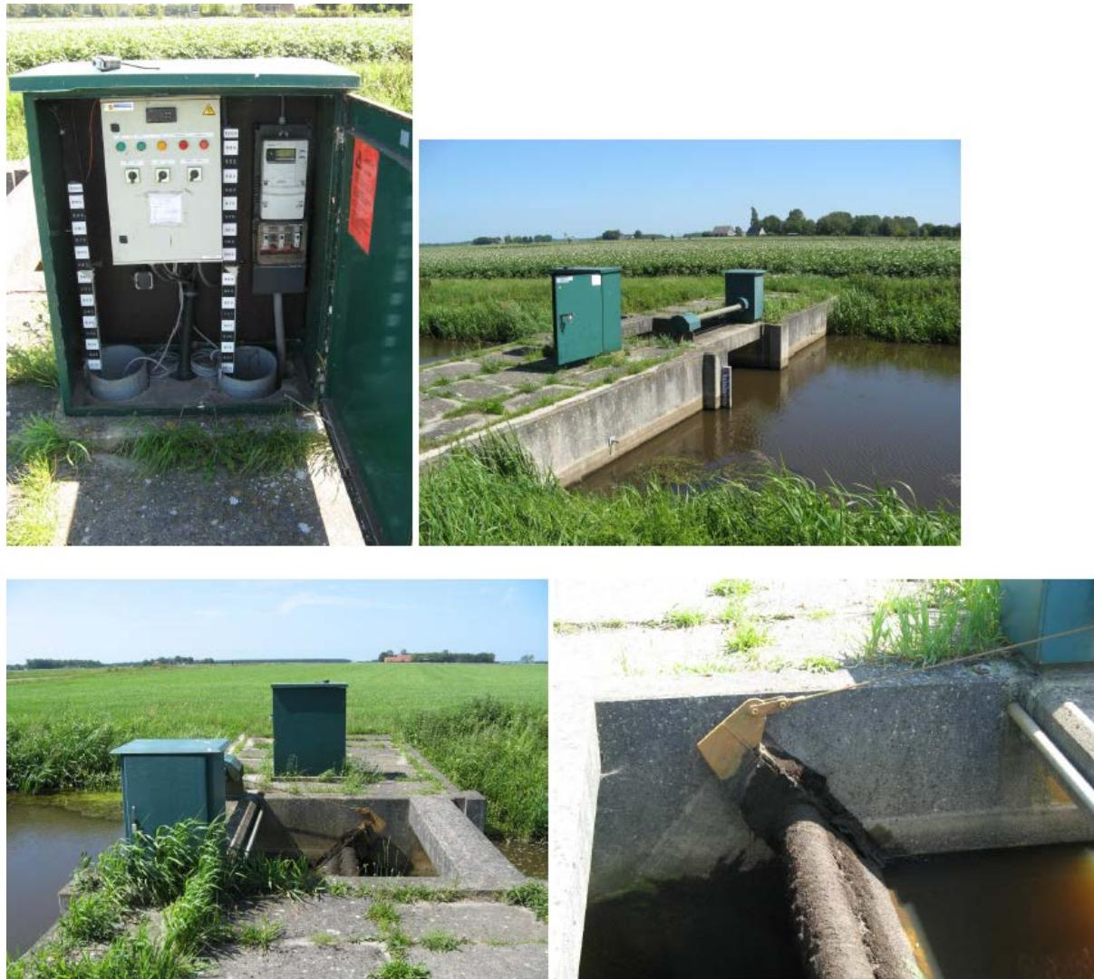
Figure 8 Weir near Nieuw Buinen with control box. The control has been upgraded from local control to remote control.
