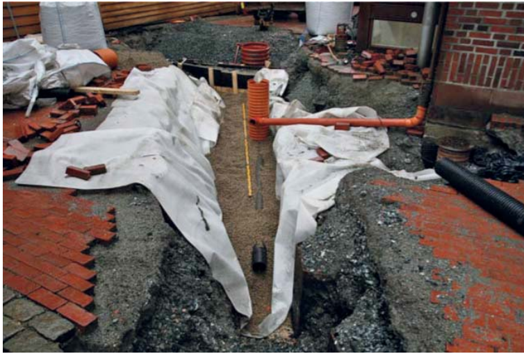
FIGURE 4. CONSTRUCTION OF SUBSURFACE INFILTRATION SYSTEM (PHOTO: R. DUNLOP, NIKU).
