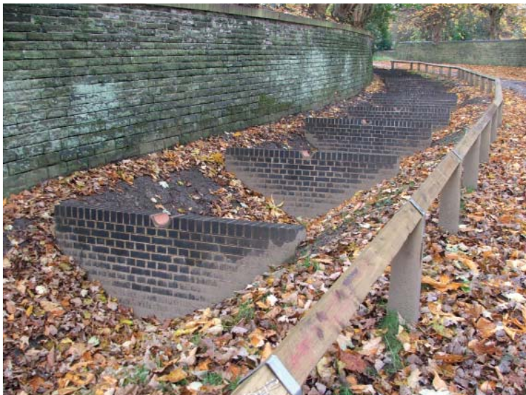
FIGURE 7. COMPLETED STEPPED TRENCH SYSTEM ON MAYFIELD ROAD
